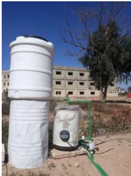
Figure 4.17: Expansion tank and water heater.
