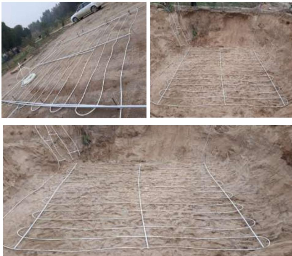
Figure 4.15 Burying the second serpentine networks at depth 2.5m.
