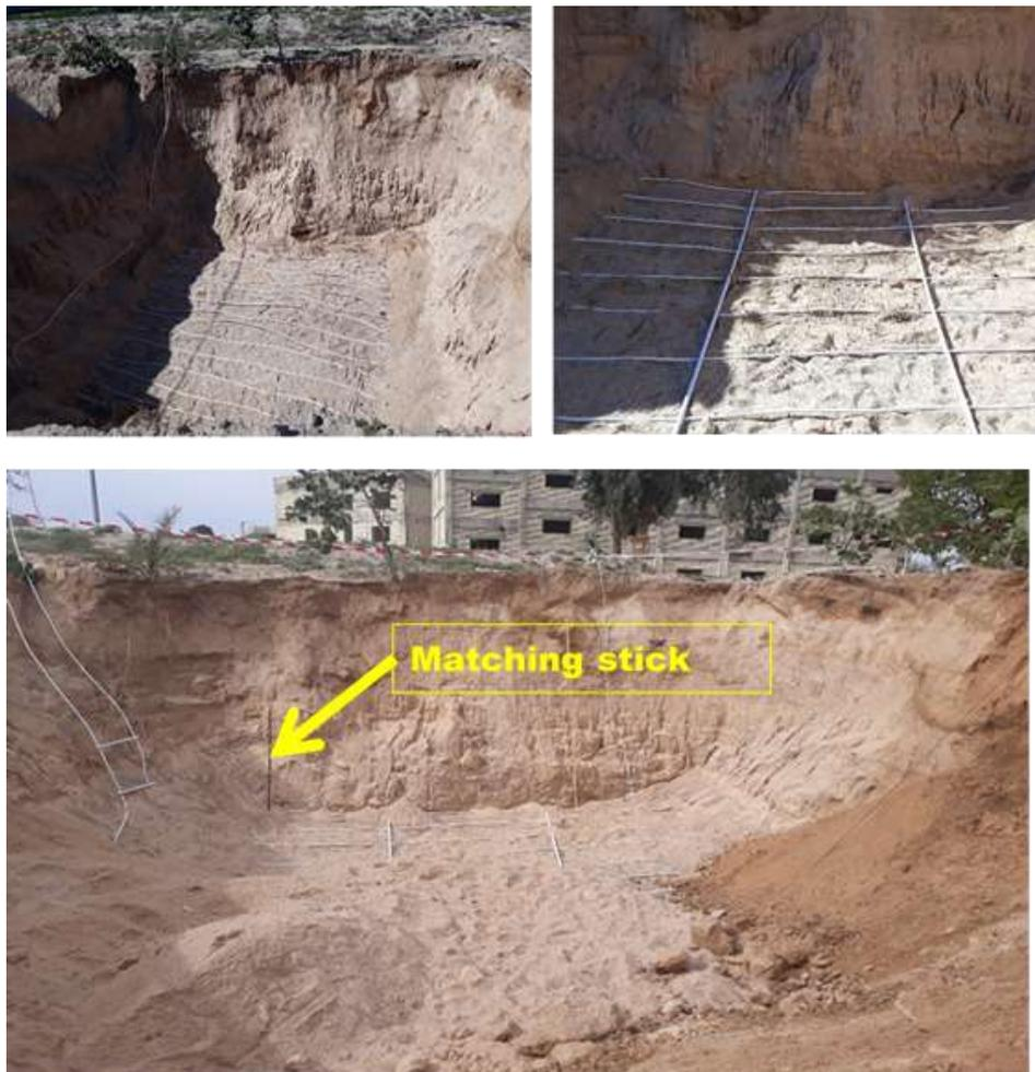
Figure 4.13 Burying the first serpentine networks at depth of 3m.
