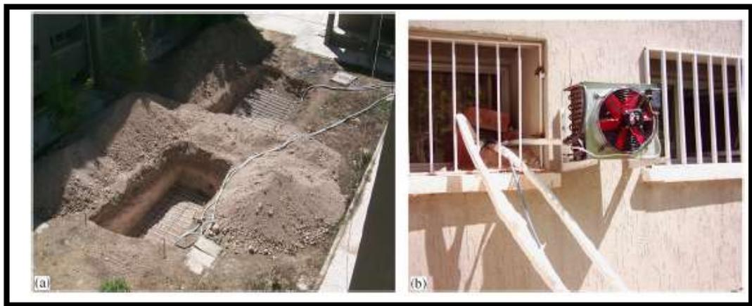
Figure. 2.1 Photographs for condenser (a) GCHP (b) ACHP[25]
