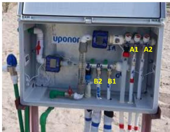
Figure 4.25 the inlet and outlet pipes mark in the system.
