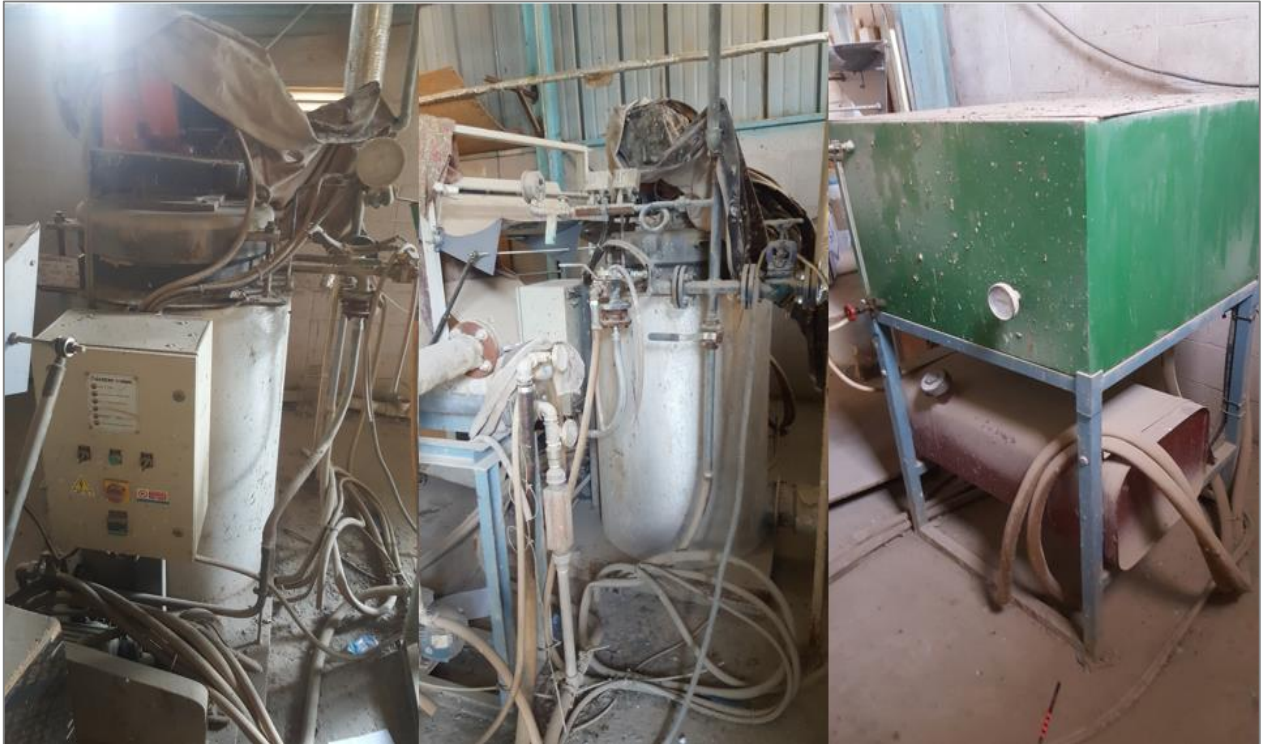
Figure 3.2: Steam Boiler before Rehabilitation
