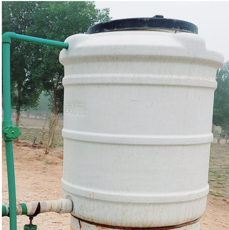
Figure. 3.4: Water tank (250) Liters.
