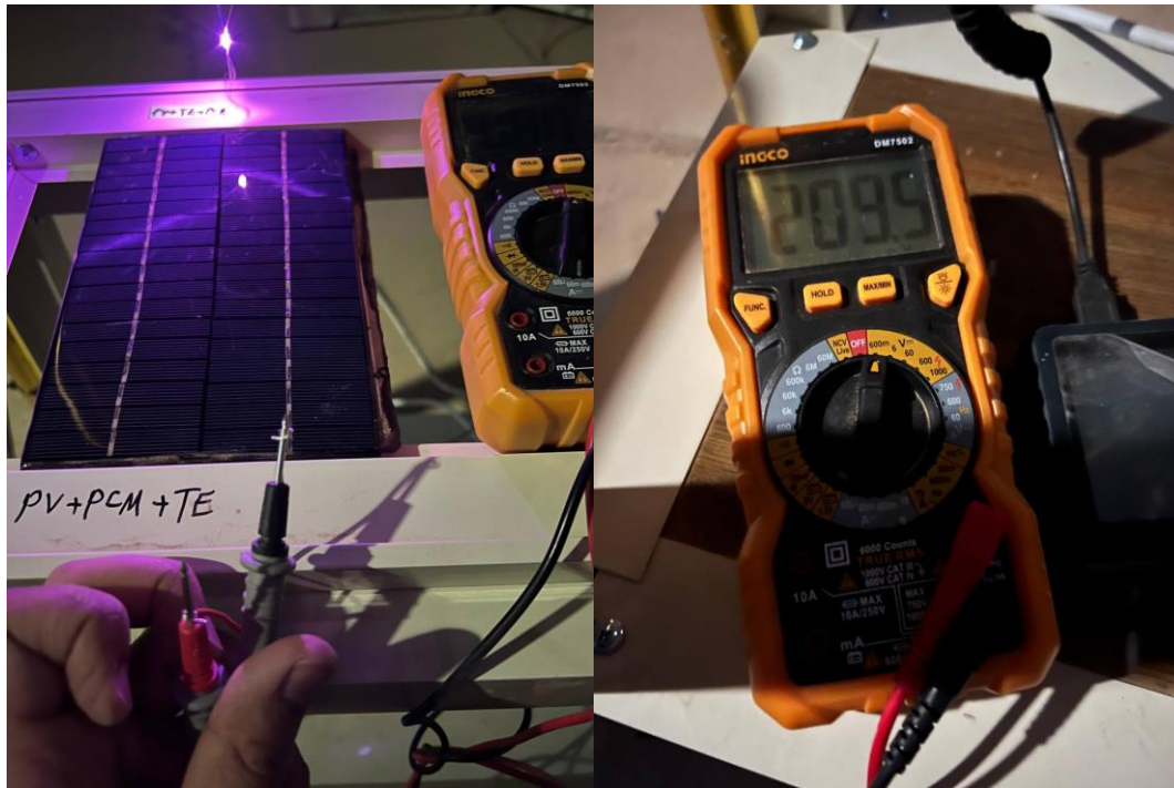
Figure (5.13) Electricity generation at night
