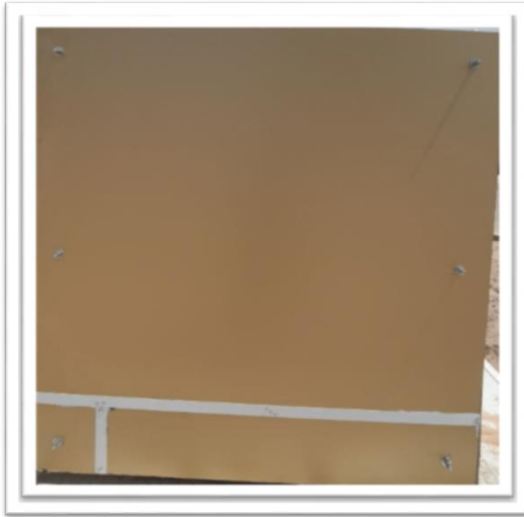
Figure . 4.3. Wall with external package (Alucobond).
