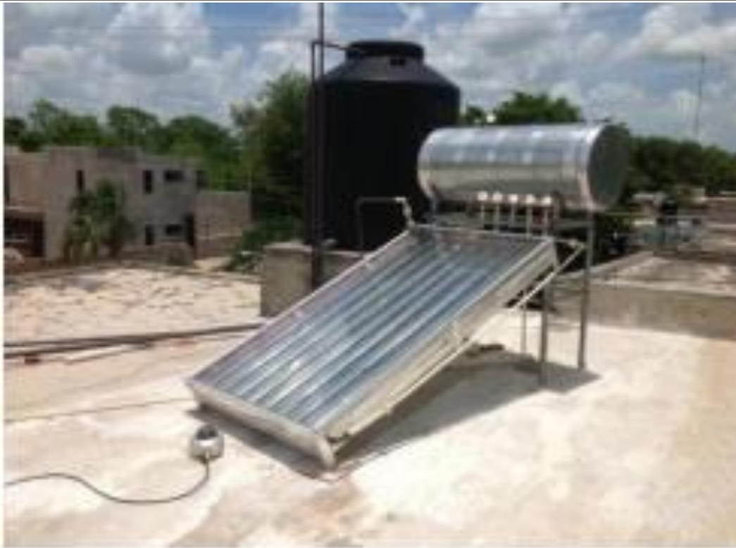
Fig. 2.17: Installation of the solar water heater [22].
