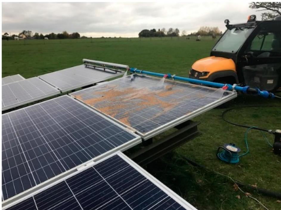
**Figure 1.8: Cleaning of PV panels [13]**
