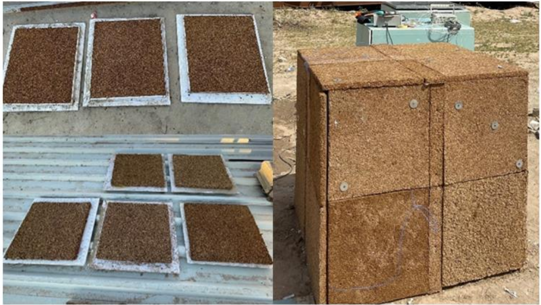
Figure 4-13 Casting and installation of the outer insulation layer
