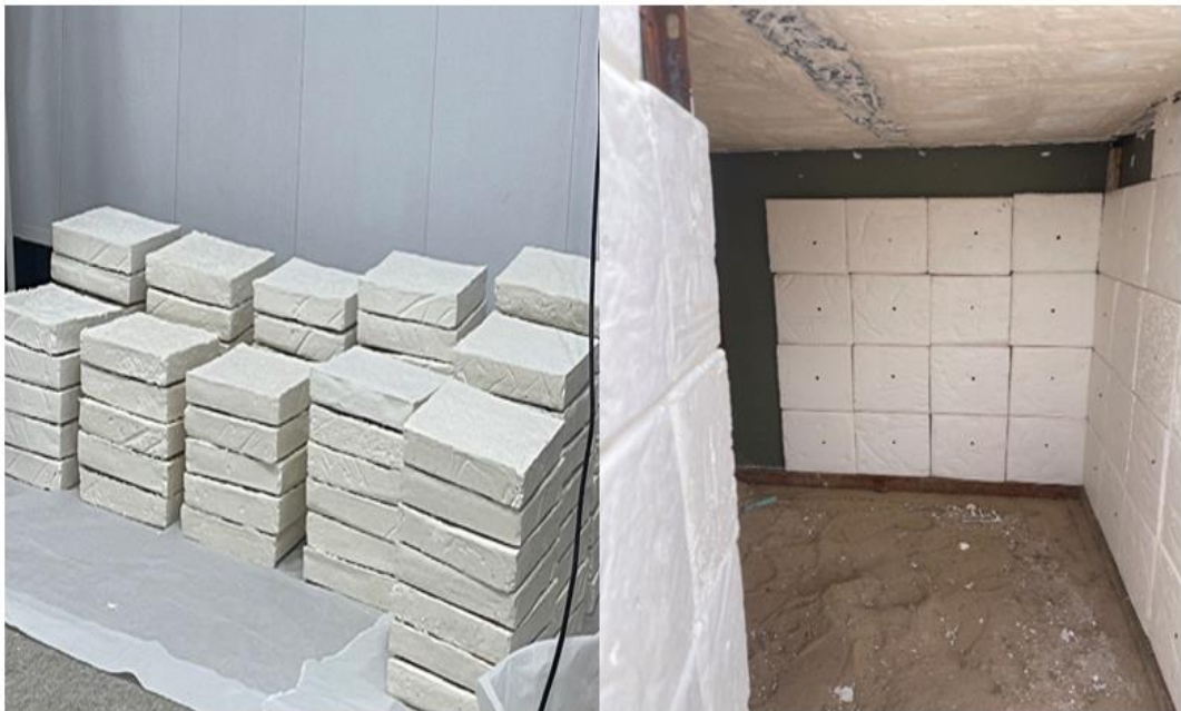
Figure 4-14 Casting and installation of the internal insulating layer
